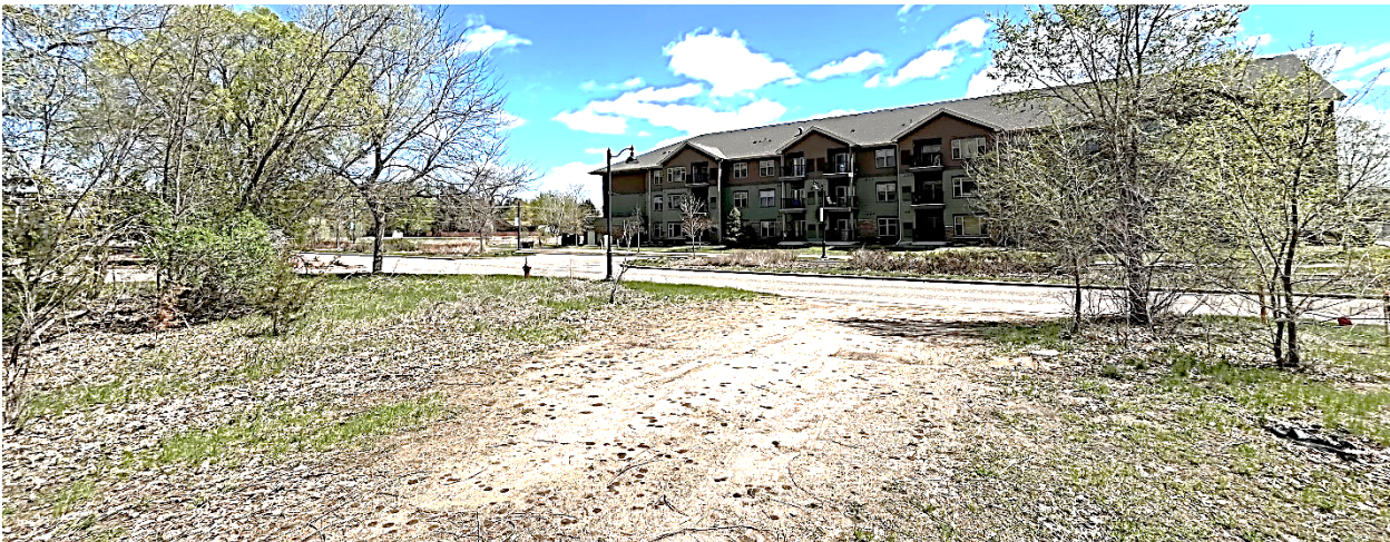
View looking east toward Balsam Apartments (Apr 30, 2026)
